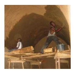
**Note:** Traditional coatings are well adapted to earth architecture, and have been used for centuries. The quality of the materials used and the skill in applying them means that they are long-lasting, even though regular maintenance is necessary.
