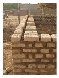
The load-bearing walls which support the vault are built of successive courses of large bricks and have a **minimum** thickness of 60 cm.
