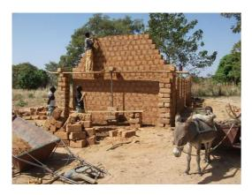
The gable walls are built with large bricks (**35 - 40 cm long**) which define the thickness of the wall. They must be built with a very slight inwards incline (of about 1 cm per metre of height).
