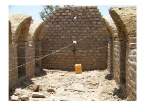
A cable, composed of 6 steel wires twisted together, is stretched from the centre of one gable wall to the opposite one at the height of the start of the vault, and in its axis. It is firmly fixed on the outside of each gable wall, and defines the axis and the curvature of the vault throughout the length of the building.
