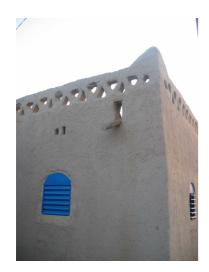
Parapets (and balustrades in the case of a flat roof terrace) should be built during the same construction phase, using mortared courses of bricks coated with the same render as the roof and walls.
