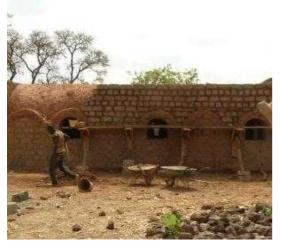
The height of the 'buttresses' can vary according to the client's wishes, but must reach at least 2/3 of the height of the vault. The best solution is to raise them to the height of the vault, thus forming a more or less flat roof terrace, because the more the loading on the vault, the stronger it is, and the flatter the roof, the lesser will be the effects of erosion during the annual rains.
