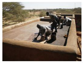
Tar-based render being applied to a roof
