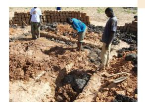
Foundation trenches for a NV will be more or less deep (30 cm - 90 cm) depending on hardness of the ground and the position of the vault - the objective being to sit the building on a sufficiently solid base.
