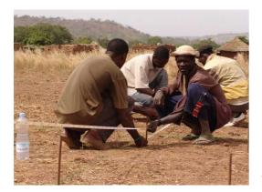
2) When laying out a NV on a limited site (for example, a specific, measured, plot of land), take care to allow for possible future extensions. The modular nature of the NV concept allows for the addition of later vaults alongside, in front, behind, or above the original one(s). This possibility should be allowed for in laying out the site at the start.
