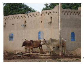
**Note:** traditional renders are well adapted to earth architecture and have been in use for gnerations. The quailty of the raw materials used combined with the traditional skills in their application mean that lasting results can be obtained, on condition that regular maintenance (from 1 to 4 years for exposed surfaces) is carried out.
