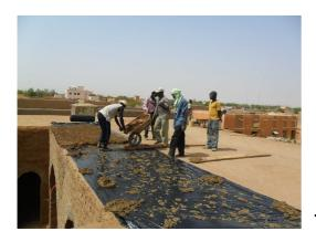
To protect the vault against rain and erosion, a tough plastic tarpaulin is laid over the roof, after it has been smoothed down and given a slight slope for draining any rain towards the gutters. The plastic tarpaulin is then itself protected with an earth mortar render of at least 5 cm thickness, using a mortar that has been enriched with waterproofing adjuvants (shea butter, other traditional 'recipes', used engine oil etc).
